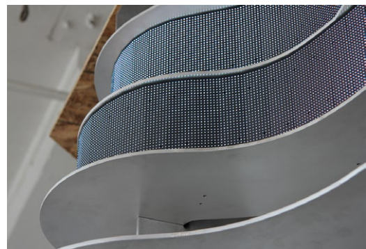
▲ The interior frame is built of aluminium in slices like this
